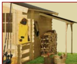
Lean to roof
